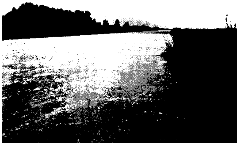
Figure 1. All-American Canal, near Calexico, California. Canal width is approximately 30 m.
