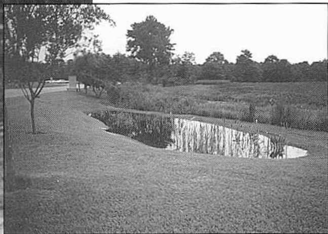
Pretreatment Sediment Basin ▲
