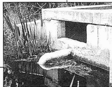
▲ Wet detention pond outfall structure.
